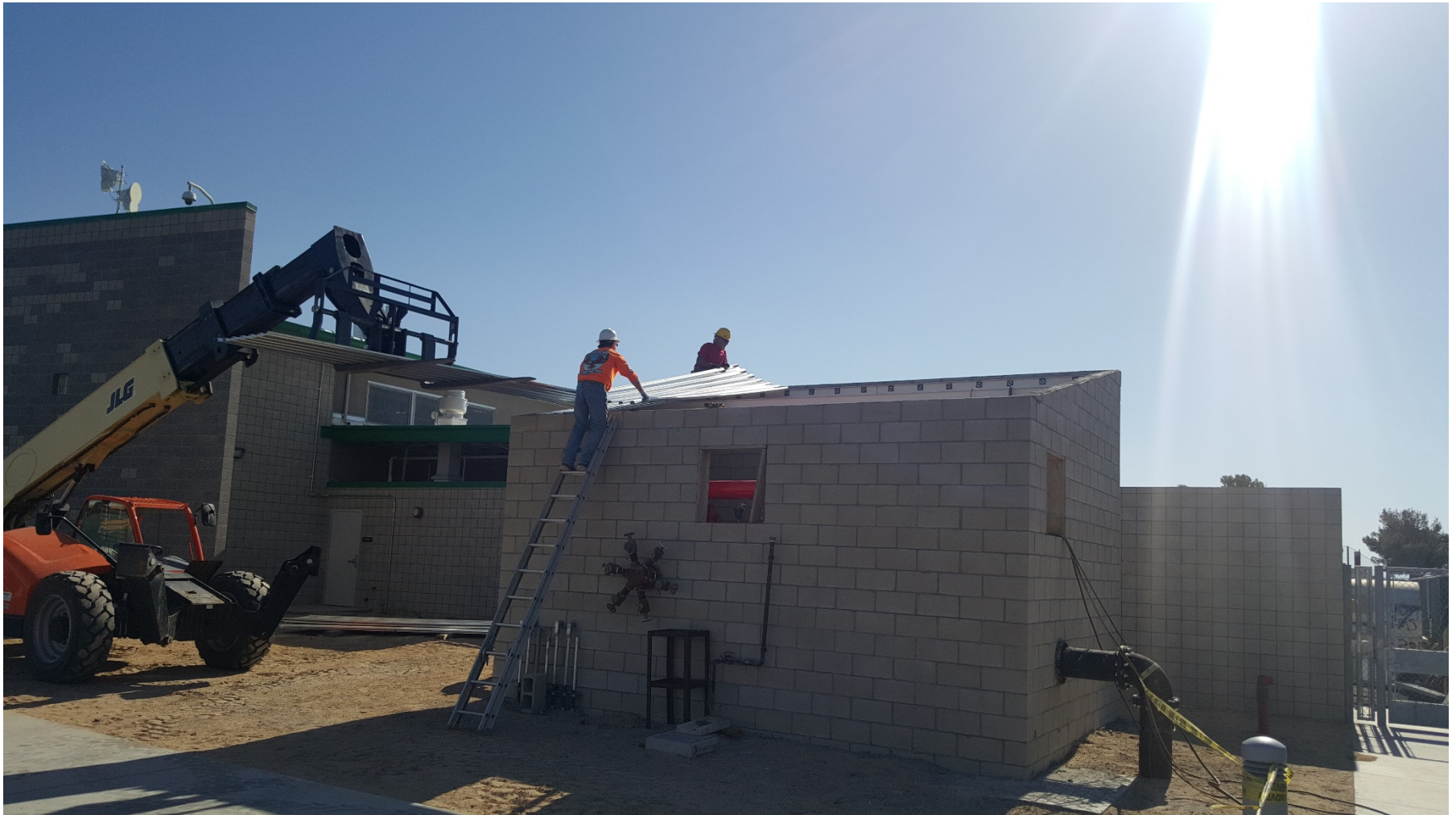
Superstructure complete for roof installation at Pump House
